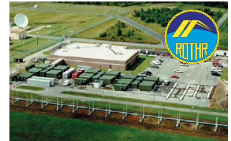
ROTHR Radar Radar Equipment Complexes
